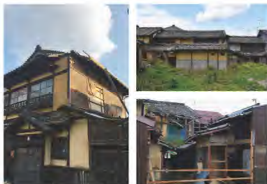
Building condition before renovation
